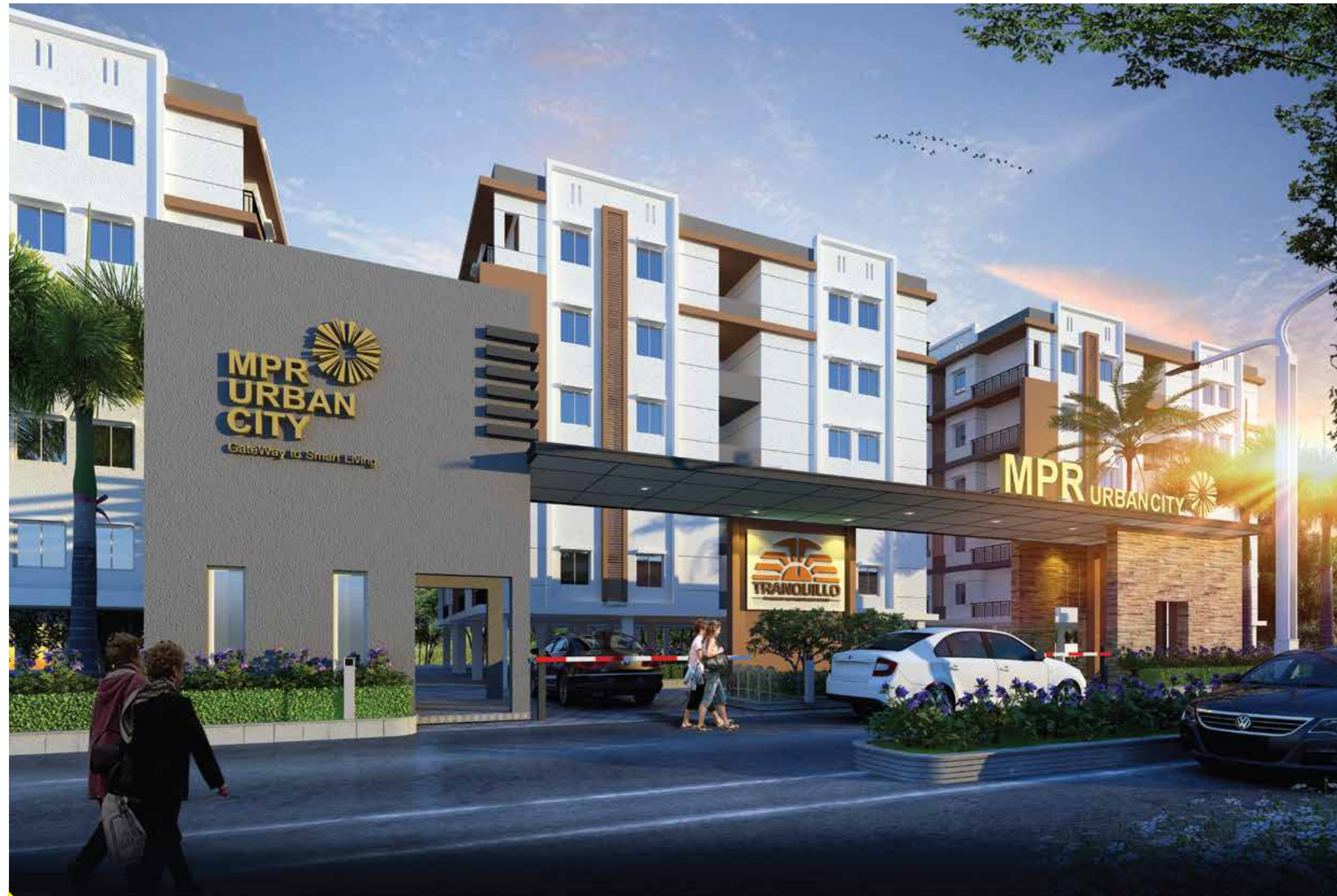
* an artistic impression of MPR Urban City grand entrance, Sapphire & Ruby Blocks view
